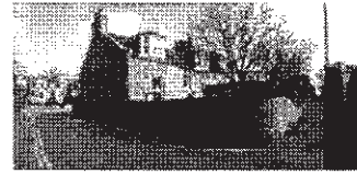
Existing view from South West
